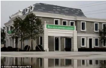
Fig.5. 2-storey building printed with a 3D printer
