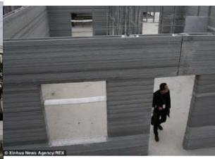
Fig.6. Printed blocks for buildings. Exhibition in the Technopark of the Chinese Province of Jiangsu
